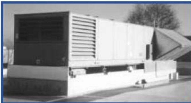
Examples of properly restrained HVAC equipment surviving the 1994 Northridge earthquake unscathed. On the left is a rooftop installation directly next door to the collapsed parking garage in Northridge. On the right is a rooftop installation across from the I-10 collapse.
