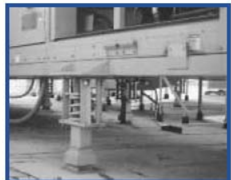
Examples of properly restrained HVAC equipment surviving the 1994 Northridge earthquake unscathed. On the left is a rooftop installation directly next door to the collapsed parking garage in Northridge. On the right is a rooftop installation across from the I-10 collapse.
